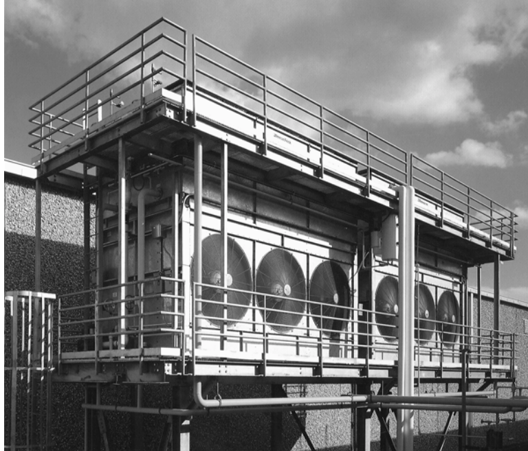
Figure 5-2: Evaporative Condenser
